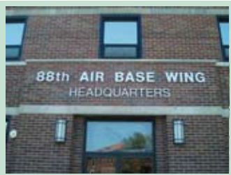
Wright-Patt Air Force Base/Dayton, Ohio-Exterior Wall Sign-Cast Metal Letters with Anodized Finish
